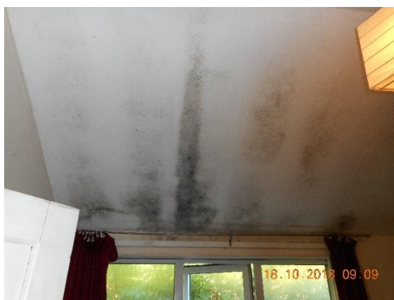
Before enforcement notice
