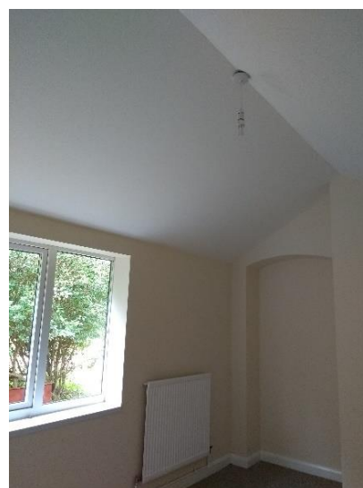
Following works required by enforcement notice
